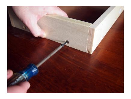
Step 6: Repeat steps 4 & 5 using C2's on the short side with 1-1/4" screws (K).
