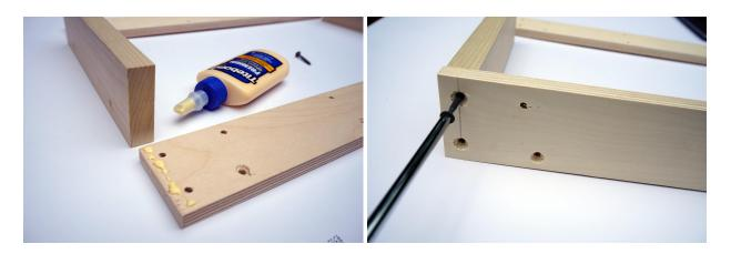
Step 3: Locate the 2 long bottom cleats (C1), two short bottom cleats (C2), 8 1" screws (J), and  $4 \cdot 1-\frac{1}{4}$ " screws (K).
